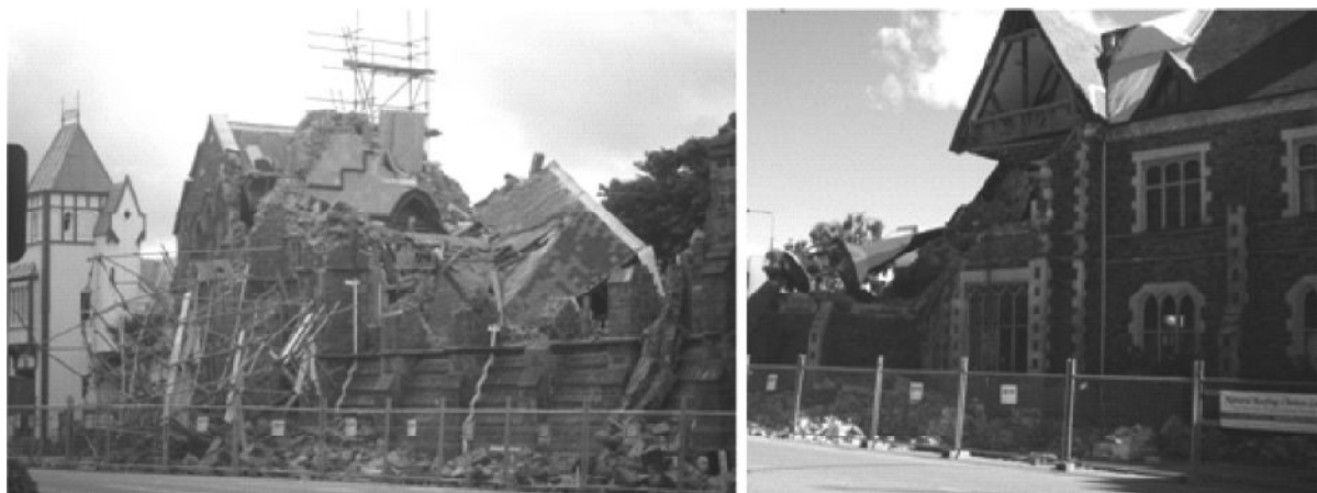
Figure 14. Collapse of URM buildings in the February 2011 earthquake.
